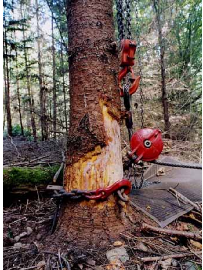
Figure 17. A piece of angle-iron keeps chain from slipping up an anchor tree when cable is tightened through the snatch block with a chain hoist. (Photo by Brian Mitchell)
