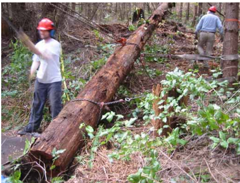
Figure 16. Nathan Gaylor pulls briskly on the chain hoist to raise the snag. (Photo by J. Azevedo)
