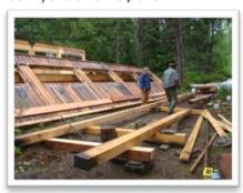
The South wall was reinforced as the North wall had been. We then lowered it onto the floor using both 1-ton hoists behind it (South side) and the 5-ton hoist to the North to pull it over gradually. The pouring rain ceased as the wall touched the floor!
