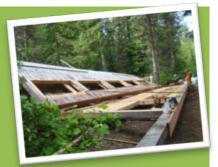
Meanwhile, once the South wall was out of the way, we began removing floorboards, carefully labeling for reconstruction ease.
