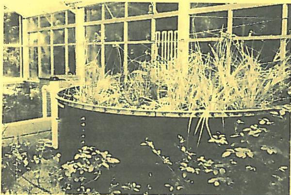
Rainwater harvesting cisterns are some of the centre's bold architectural statements that show attention to the way they use the land. Roofs have been sloped to capture maximum water, as well as for sunlight exposure. Islandwood expects to produce at least 50% of its energy needs through photovoltaic panels. Photo: Meg Holden.
