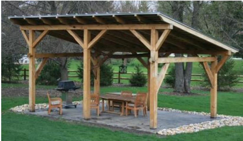
Figure 6: An example of a wood shelter that could be used in the backcountry campsite learning space. Our recommendation is to create a similar structure without the concrete base. Retrieved from: http://www.trilliumdell.com/timber-frame-pergolas-porches-pavilions.html
