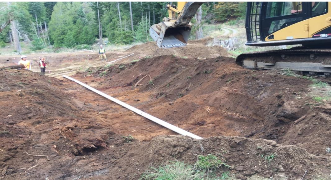
Upper left: volunteers raking out the wetland rim to ensure consistent elevations. Lower left: extending the classroom's perimeter drainpipe into the wetland
