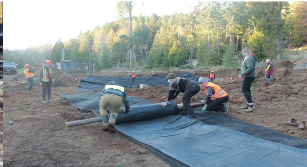
Upper right: basin complete, one last centre depth check Lower right: Volunteers unravel and install the three layers of geotextile and pond liner
