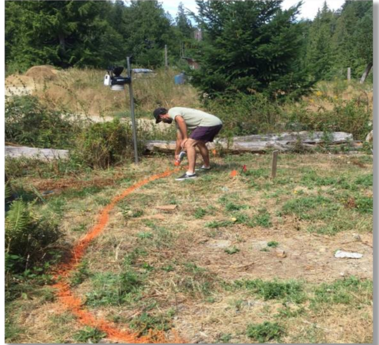
Figure 11: Spraying out a wetland footprint
