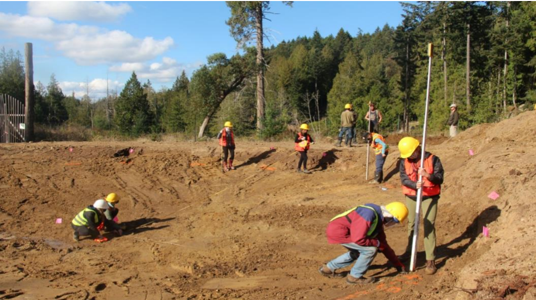
Upper left: volunteers raking out the wetland rim to ensure consistent elevations. Lower left: extending the classroom's perimeter drainpipe into the wetland
