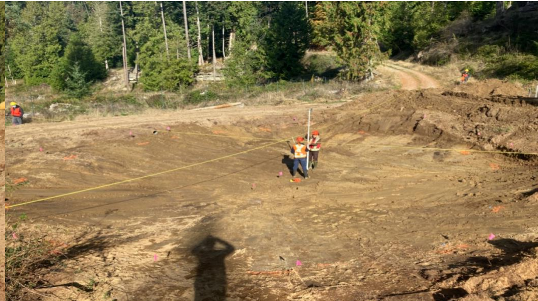
Upper right: basin complete, one last centre depth check Lower right: Volunteers unravel and install the three layers of geotextile and pond liner
