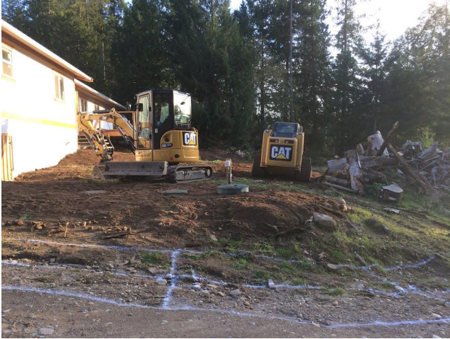
Figure 7.2.2 and 7.2.3: Excavator levels out the top of site A (left); Excavator digs out and places large rocks in the bioswale trench (right)
