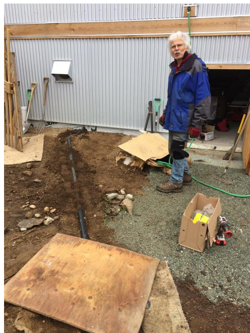
Figure 7.3.4: Creation of the branched greywater system to the greywater garden bed. Piping is connected to the Project Centre greywater outlet (top left). Trenches dug allot branched greywatersystem to water fruit tree mounds (top right). Volunteer crew stands proudly by their work (bottom right)
