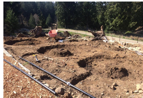
Figure 7.3.3: Creation of the bioswale from recontouring to planting. Water is collected from part of the roof and run-off from the above parking lot (top left). Excavator recontours bioswale by digging out a trench and placing large stones to create bioswale tiers (top right). GCA intern Sadie checks out the gravel filled bioswale (bottom left). Volunteers plant willow to stabilize the bioswale bank and place burlap sacks over planted areas (bottom right).
