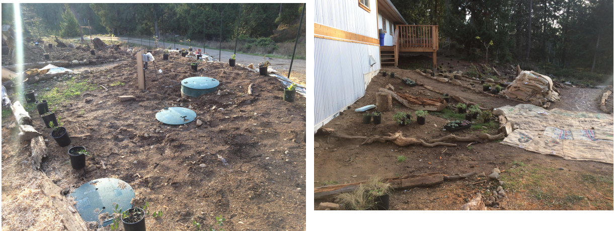
Figure 7.3.5: Potted plants are placed during the first weekend of restoration planting at site A
