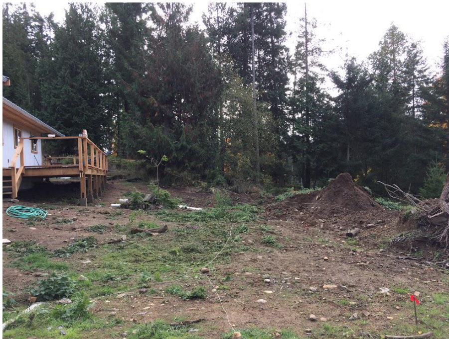
Figure 7.2.1: String marks the pathway layout near the Project Centre deck, October 2019
