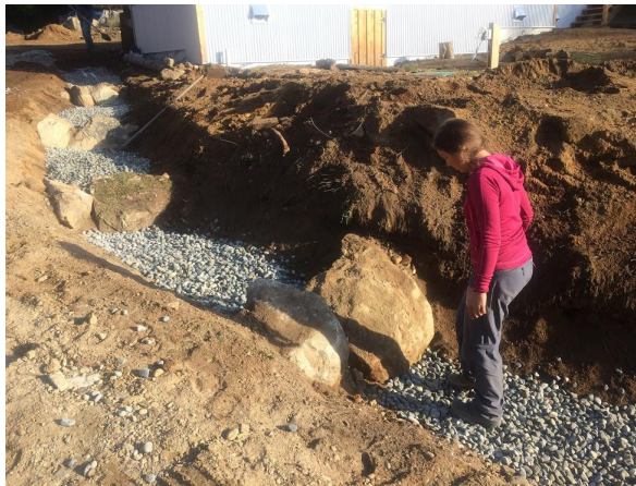
Figure 7.3.3: Creation of the bioswale from recontouring to planting. Water is collected from part of the roof and run-off from the above parking lot (top left). Excavator recontours bioswale by digging out a trench and placing large stones to create bioswale tiers (top right). GCA intern Sadie checks out the gravel filled bioswale (bottom left). Volunteers plant willow to stabilize the bioswale bank and place burlap sacks over planted areas (bottom right).
