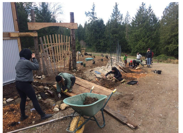
Figure 7.3.3: Creation of the bioswale from recontouring to planting. Water is collected from part of the roof and run-off from the above parking lot (top left). Excavator recontours bioswale by digging out a trench and placing large stones to create bioswale tiers (top right). GCA intern Sadie checks out the gravel filled bioswale (bottom left). Volunteers plant willow to stabilize the bioswale bank and place burlap sacks over planted areas (bottom right).
