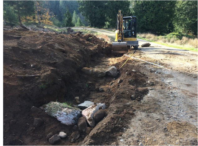
Figure 7.2.2 and 7.2.3: Excavator levels out the top of site A (left); Excavator digs out and places large rocks in the bioswale trench (right)
