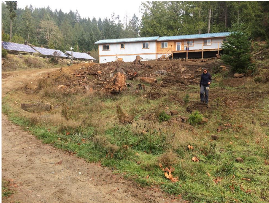
Figure 7.2.4: After machine work is completed Site A is recontoured and coarse woody debris is redistributed
