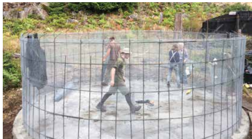
Ferrocement cistern, mid-construction in summer 2019.
