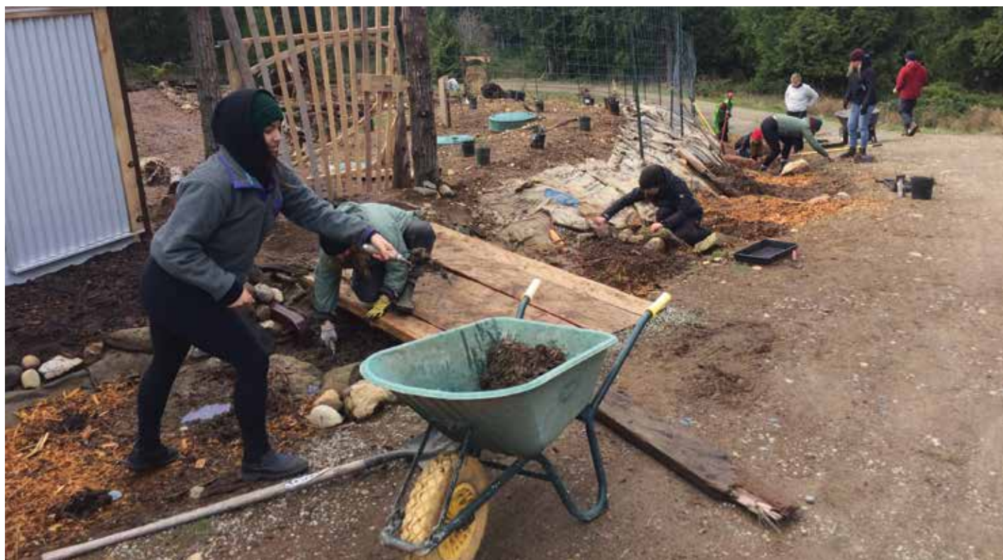
UVic students help establish native species to filter runoff in the Program Centre bioswale in February 2020.
