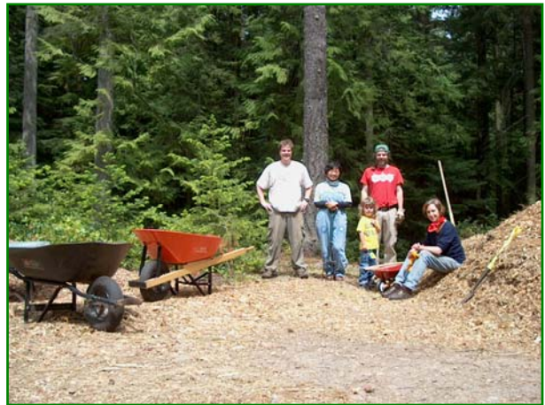
Preventing root damage to trees by "re-surfacing" trail with wood chips in the Pebble Beach Reserve
