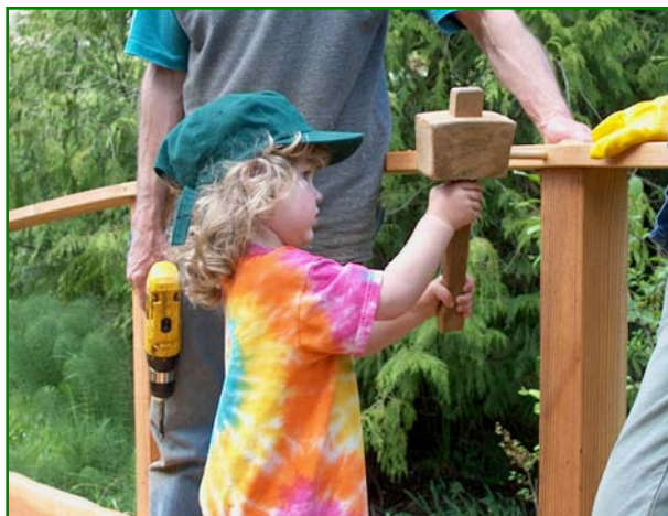
Building a bridge out of local wood (Laughlin Lake) Odin Scholz
