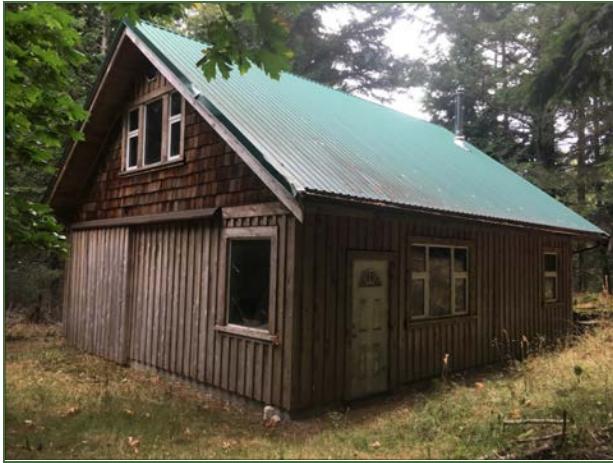
Photo 1 - Detached Garage (unserviced)
